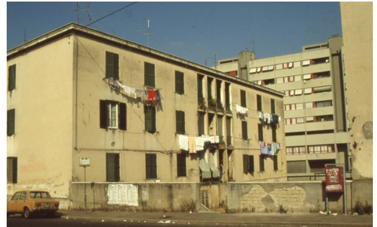
Tiburtino III demolished
